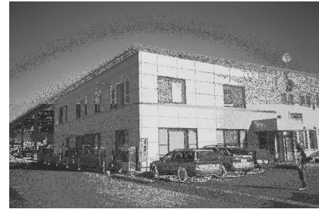
Fig. 4, ALPOLIC project where the survey was held
